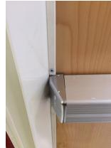
Bend fixing strip and place in corner with wider section on the door side.
